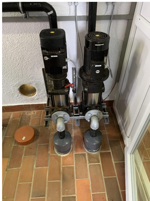
Rentvandspumper
